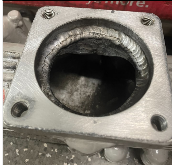
Figure 2: Crack through internal fillet weld
